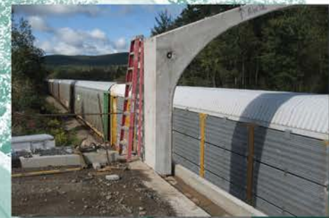
Work progressing along an active railway line
