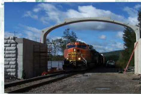
Construction was phased to ensure the railway could still operate
