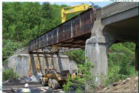
Demolition of the existing bridge.
