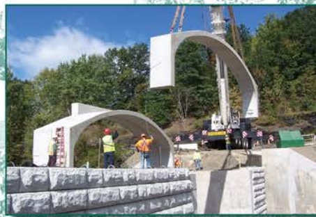
Placing the pre-cast concrete arches
